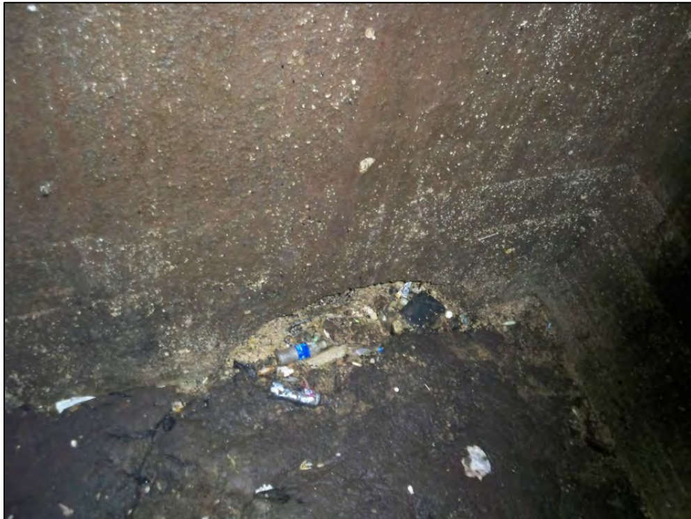
Figure 6: Manhole 14L013 Junction Box Crossing
