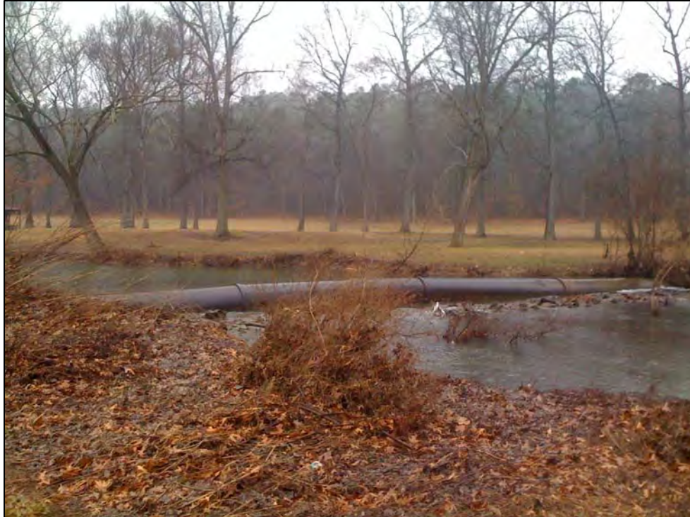
Figure 5: Hindman Park Aerial Crossing
