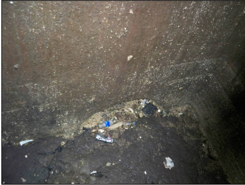
Figure 4.2: Manhole 4L013 Junction Box Crossing
