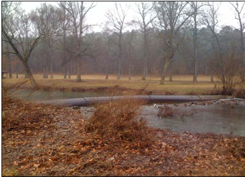
Figure 4.1: Hindman Park Aerial Crossing
