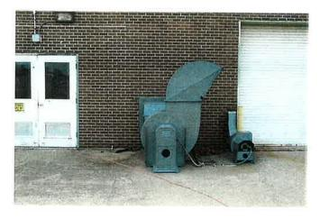
Figure 31. East side dry well and wet well blowers.
