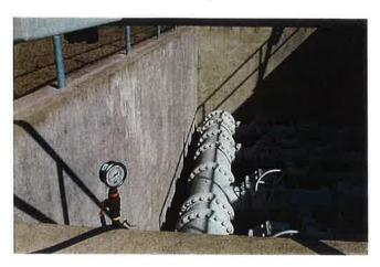
Figure 42. Pump header pressure gauge.
