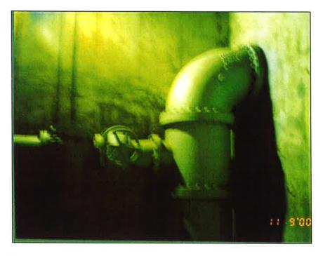
Figure 27. Drain/return line into wet wells off of discharge manifold.
