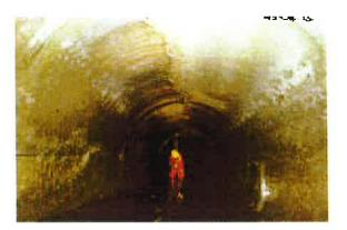
**Fracture Longitudinal.** When a crack becomes open on the pipe wall and the pieces are all still in place. The defect runs approximately along the axis of the sewer.
