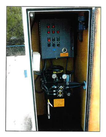
Figure 6. Grinder control panel.
