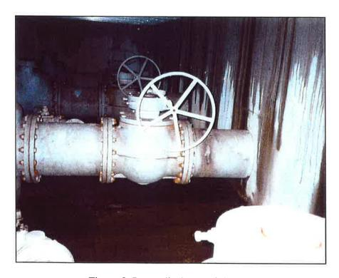
Figure 8. Pump discharge piping in dry well.
