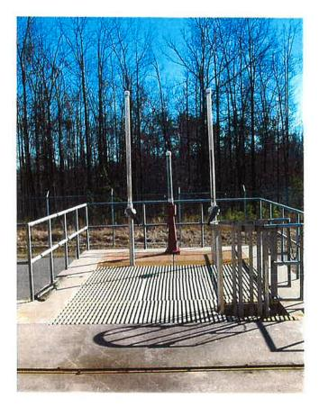
Figure 43. Fiberglass grating over influent and grinders
