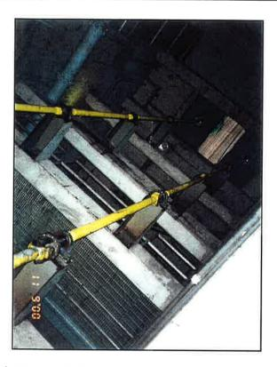
Figure 20. Extended drive shafts for Fairbanks Morse pumps.
