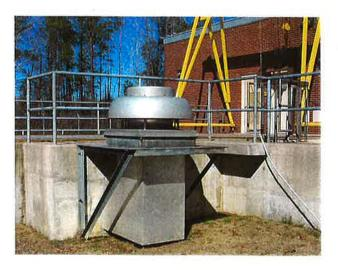
Figure 44. Wet well exhaust fan.
