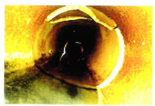
**Broken**. Pieces of the pipe are noticeably displaced. Some pieces could be missing. A hole in the fabric of the sewer is also classified as "broken." A chipped pipe is not classified as broken.
