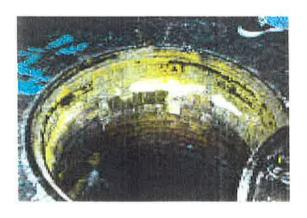
FIGURE A-6 LOOSE AND MISSING MANHOLE BRICKS
