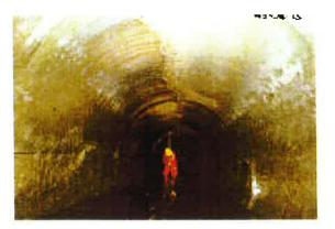
**Fracture Multiple.** When a crack becomes open on the pipe wall and the pieces are all still in place. The defect runs approximately along the axis of the sewer. Combination of both longitudinal and circumferetial (that cannot be easily identified and coded as either one).
