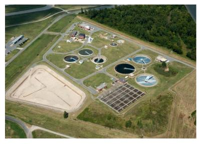
Rock enters the plant via three 60-inch diameter gravity sewer lines at an average depth of 30 feet below ground and requires the pumping or lifting of the sewage to the surface.
