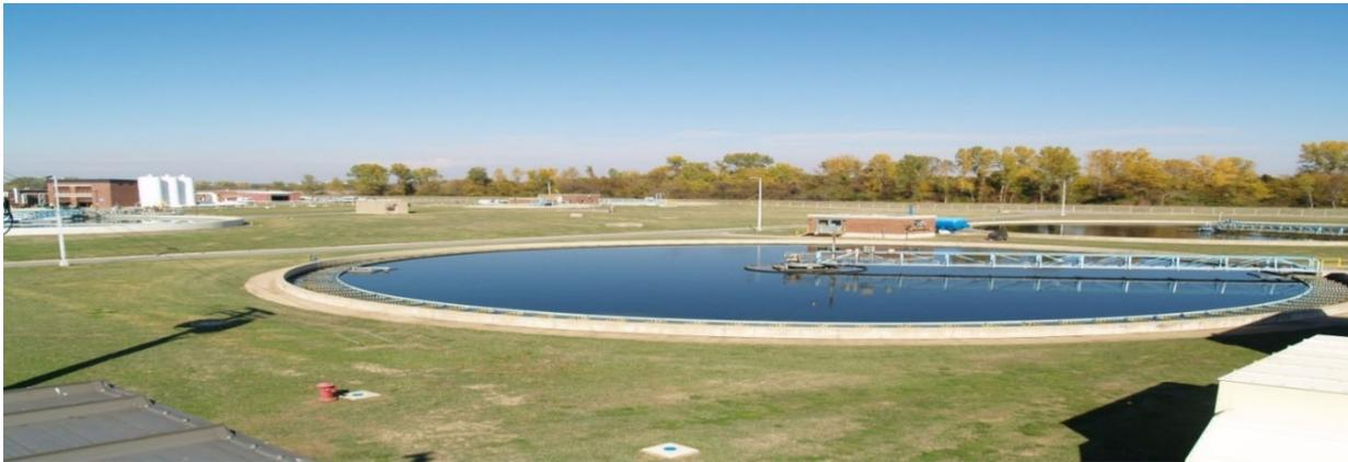
The Fourche Creek Water Reclamation Facility (FCWRF) has been providing wastewater treatment to the Fourche Creek Valley since 1983 when it was placed in service at a cost of \$19.6 million. The step-feed activated sludge process was brought online in 1989 at a cost of \$9 million. The FCWRF is also a two-stage, or secondary treatment facility. It has a rated biological treatment capacity of 16 MGD. The plant's annual average dry weather influent sewage flow is 12 MGD.
